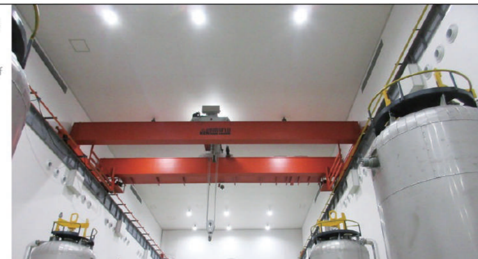
洁净防爆全自动起重 机 Clean explosion-proof full-automatic crane
