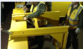
Stop hook bracket installation
