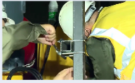
Installation of the trolley conductor bracket
