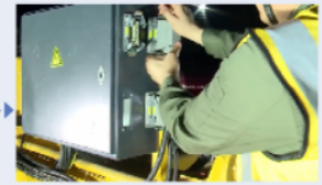
Installation of aviation plug in trolley terminal box
