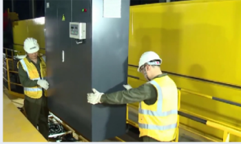
Installation of electric cabinet and resistor
