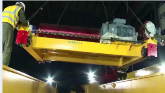
Installation of the trolley conductor bracket
