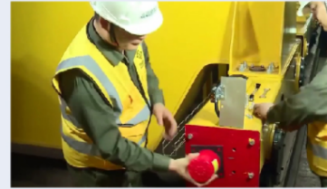
Installation of buffer
